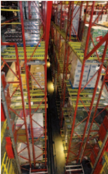
REWE impressive high-rack warehouse
